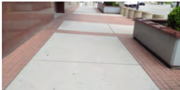
Standard concrete with brick highlights paving pattern
